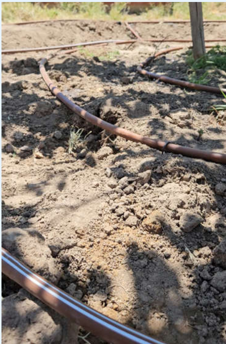
Drip line dumping water right at the trunk
